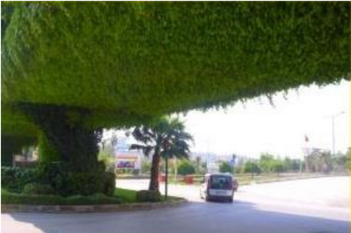
Foto 1. An example applied to a highway overpass.
