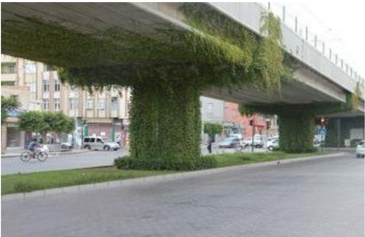
Foto 2. A developing example applied to a highway overpass.
